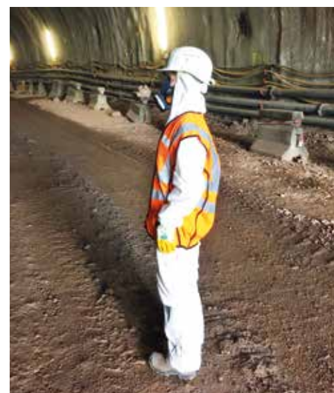
Bilder © ARGE Tunnel Brandberg
